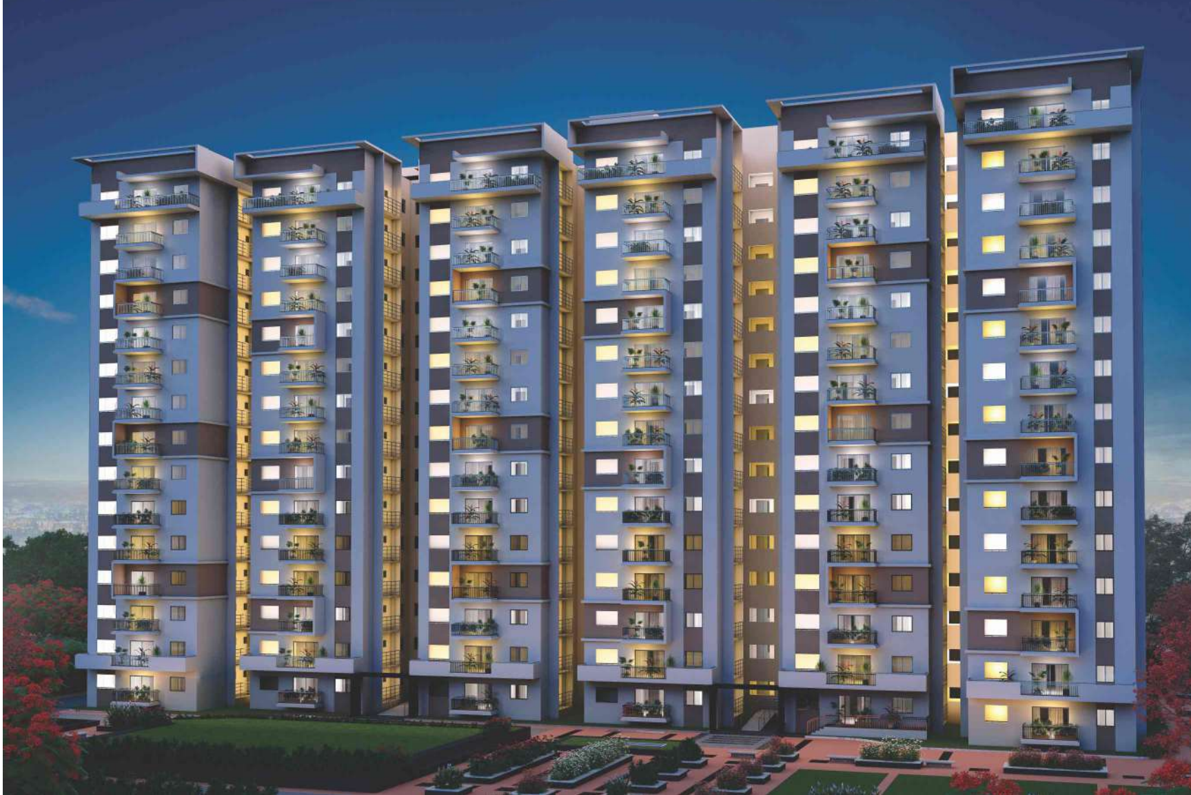
West side view
