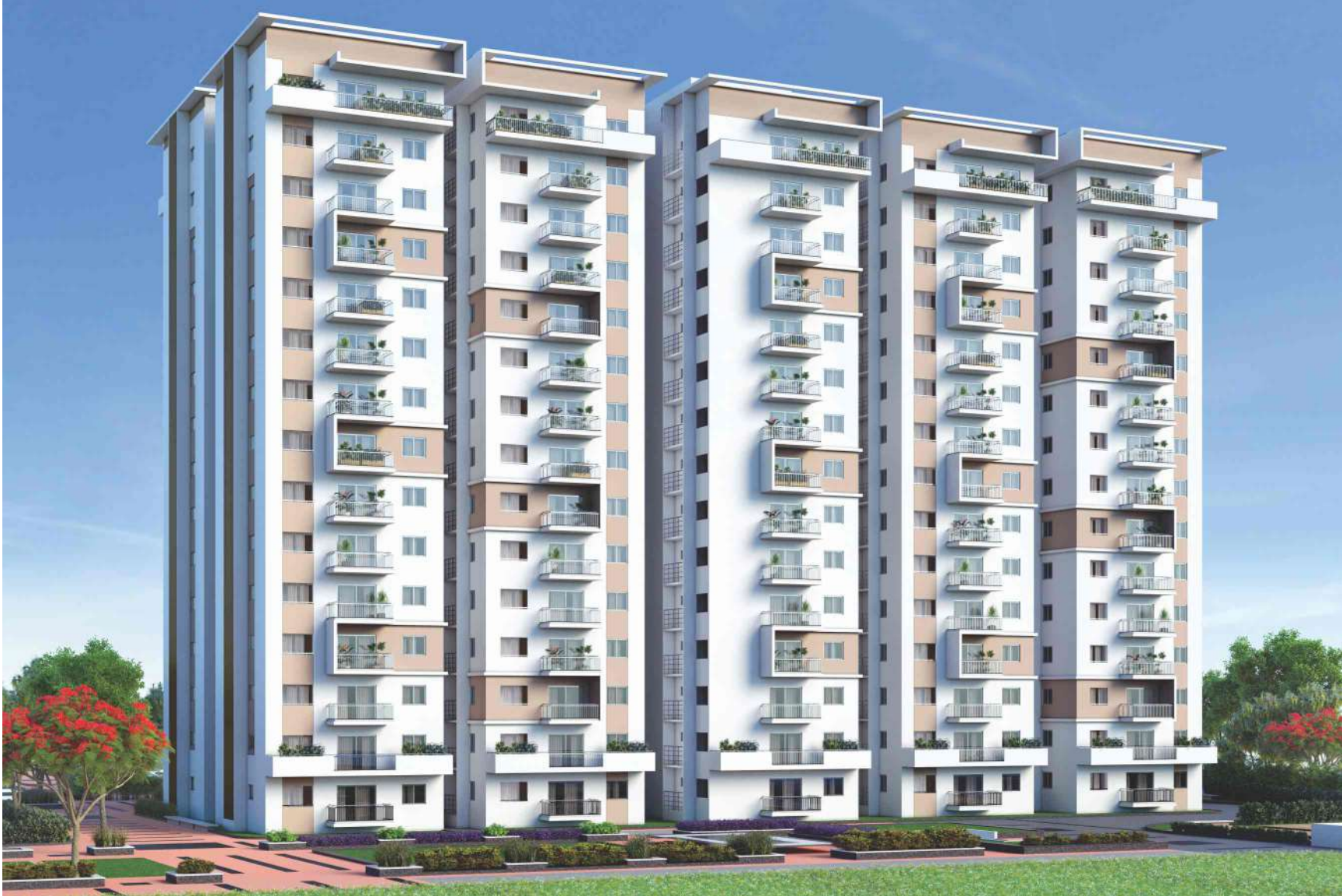
West side view
